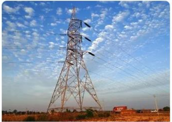
Field power cable
