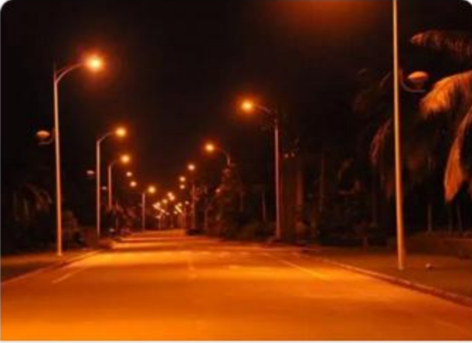
Street lamp cable maintenance
